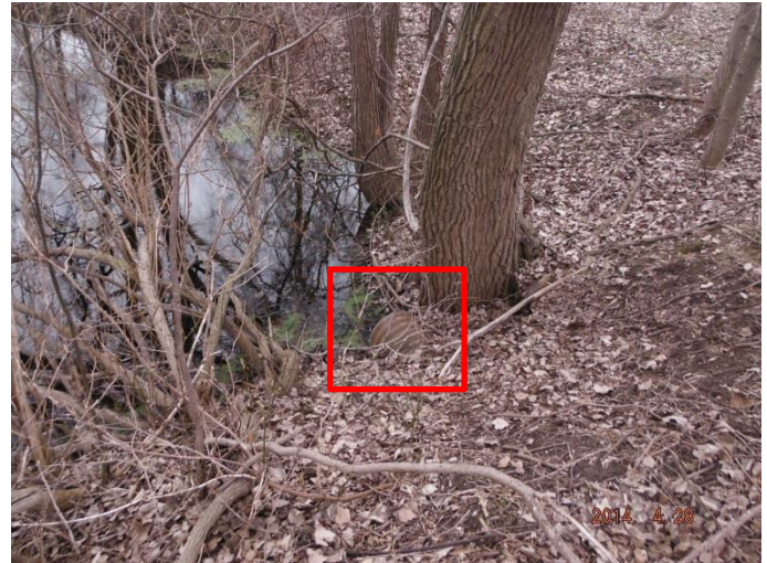
Photograph 4. ↑ Location of culvert on east side of pond.
